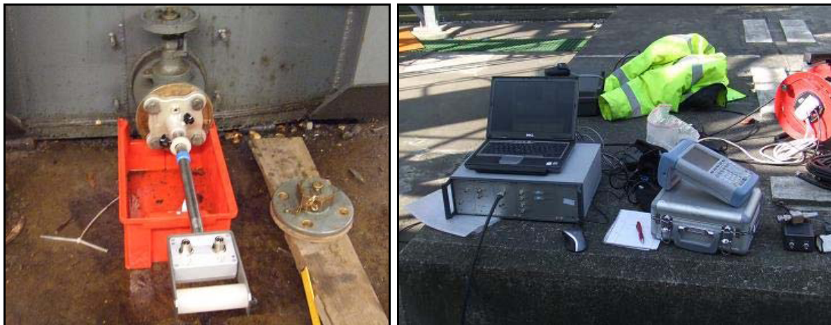
Figure 15 UHF drain valve sensor (left) and LDS-6/UHF measuring system (right)
